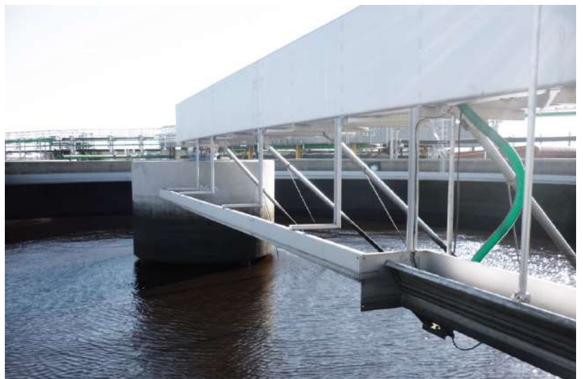
Scum flows into the channel over an adjustable flap
