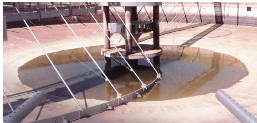
Circular scraper with dragged scraper blades
