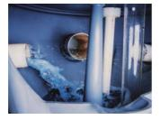
A traditional gravity line carries wastewater from a customer's home to an Airvac valve pit package.
