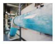
Wastewater travels at 15 to 18 fps in a vacuum main, which is laid in a sawtooth fashion to ensure adequate vacuum levels at the end of each line.
