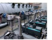
At the vacuum station, Vacuum pumps cycle on and off as needed to maintain a constant level of vacuum on
