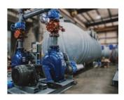
Sewage pumps then transfer the sewage to the treatment plant via a force main.
