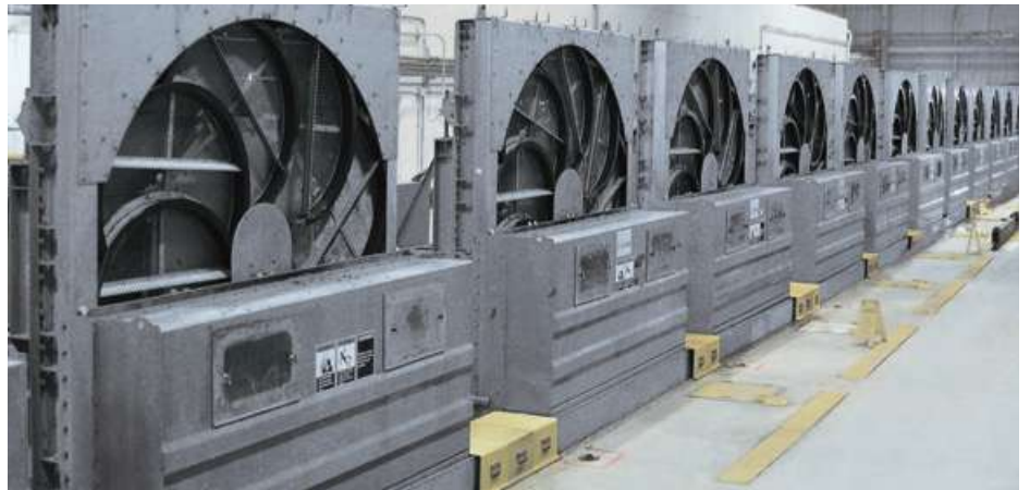
DC Nuclear Power Plant in the USA: Row of 15 Geiger MultiDisc® Screens
